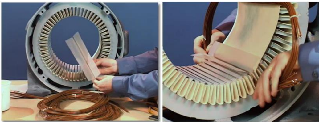
Figure 28: The process of coil insertion using scuff paper
